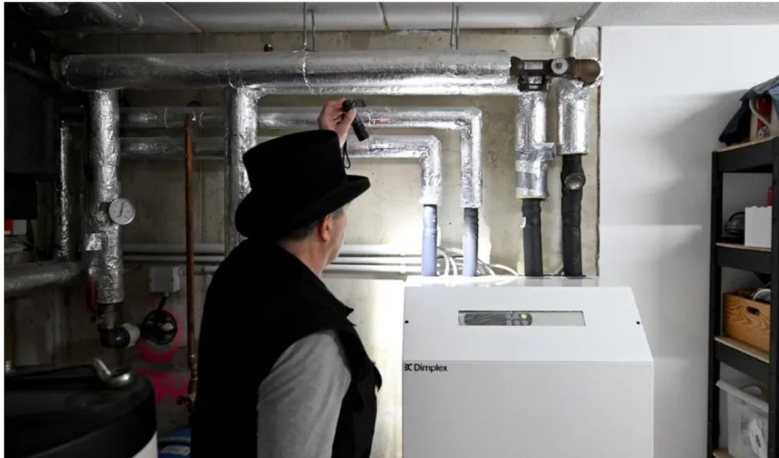
Chimney sweep Udo Löbel inspects a water-to-water heat pump with a well in the basement of a detached house in Munich on Dec. 13, 2023. (Felix Hörhager/picture alliance via Getty Images)
